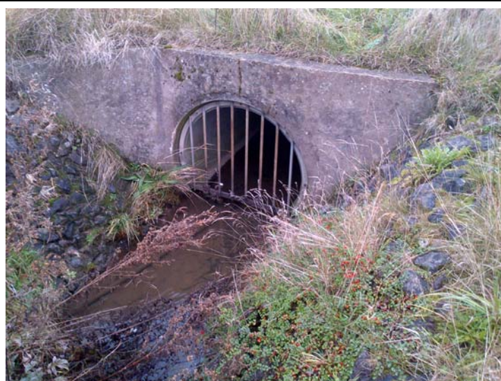
Figure 4-1: 1300mm diameter culvert entrance
